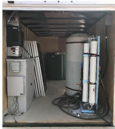
Grid + solar PV
